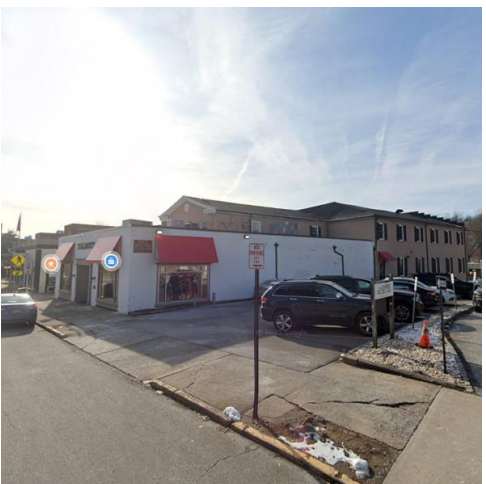
4 CLOTHING STORE/ OFFICES BUILDING
