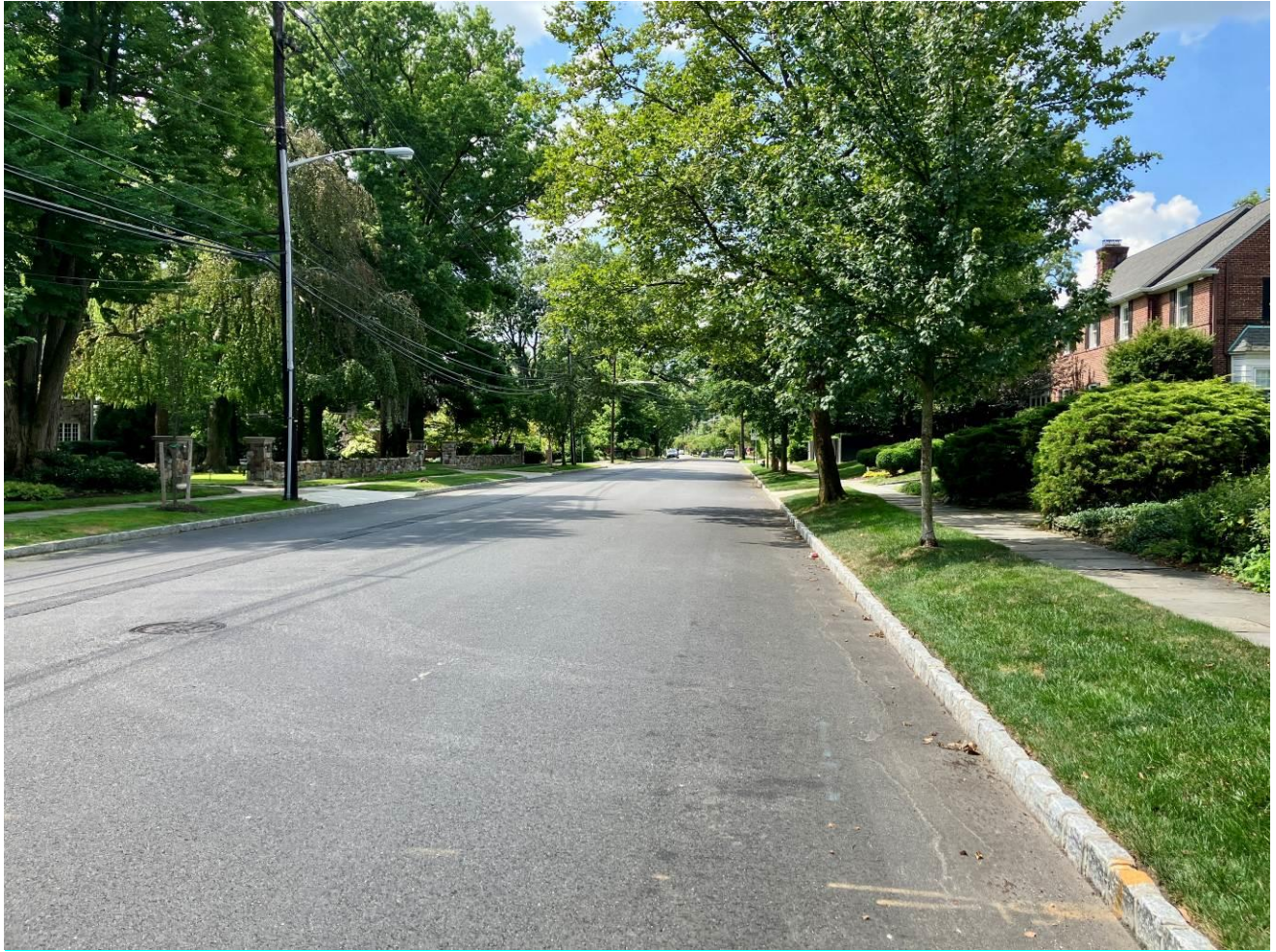
Figure 7 View looking south along Park Street, between Buckingham Road and Inwood Avenue.
