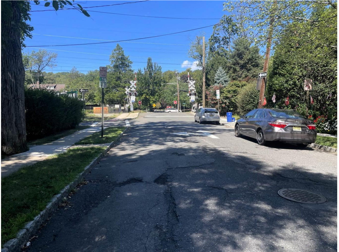
Figure 6 View looking northwest along Laurel Place towards the railroad crossing.
