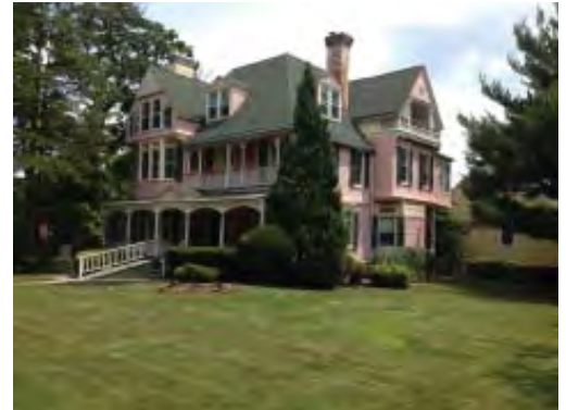
Figure 3.3.b: Historic building on North Mountain Avenue
