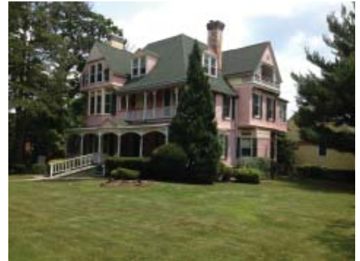
Figure 3.3.b: Historic building on North Mountain Avenue
