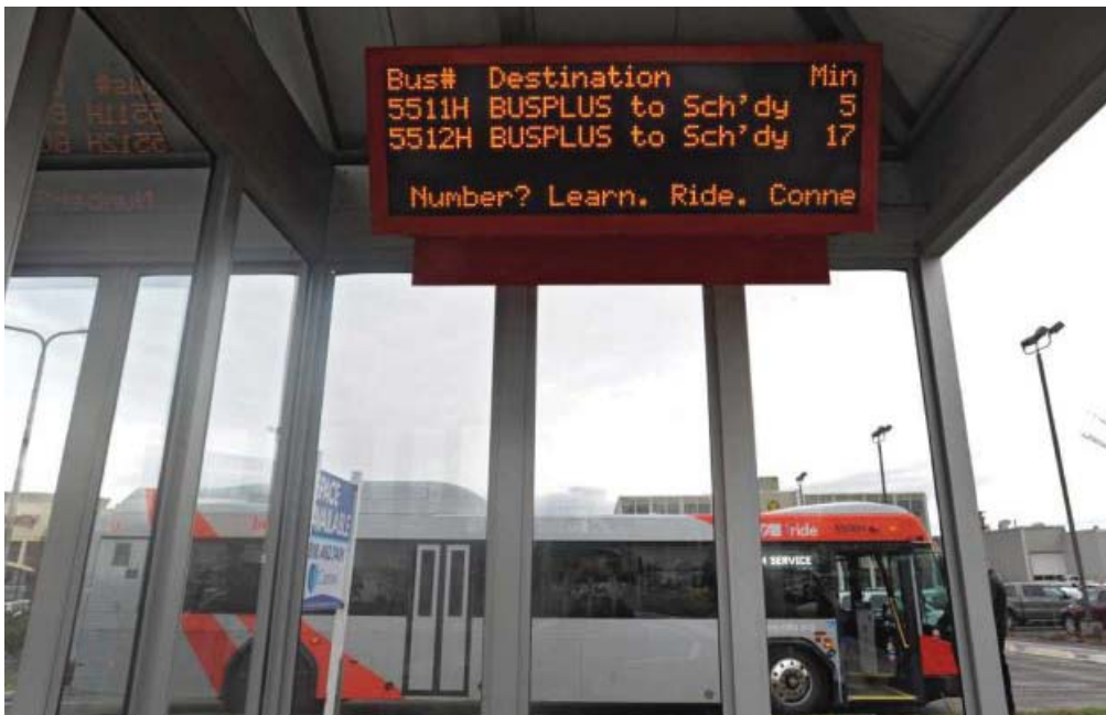
Enhanced bus stop with amenities for passengers in Albany, NY.
