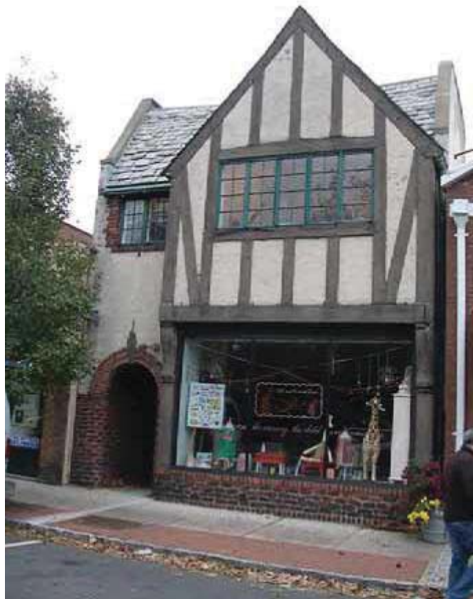
Figure 3.5.c: Watchung Plaza Key Historic Building
