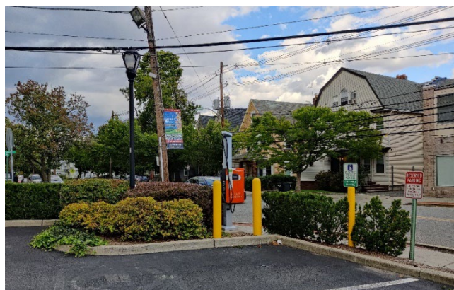
Figure 2.7c: DC Fast Charging station at local retail center.
