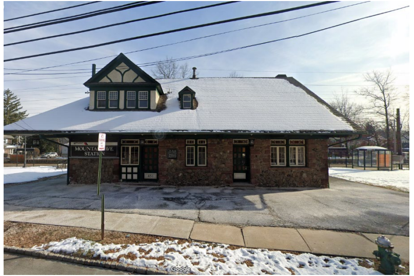
Figure 19: Mountain Avenue Train Station.
