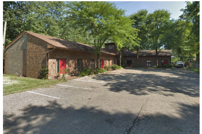
Figure 26: Office building on Beldin Place.
