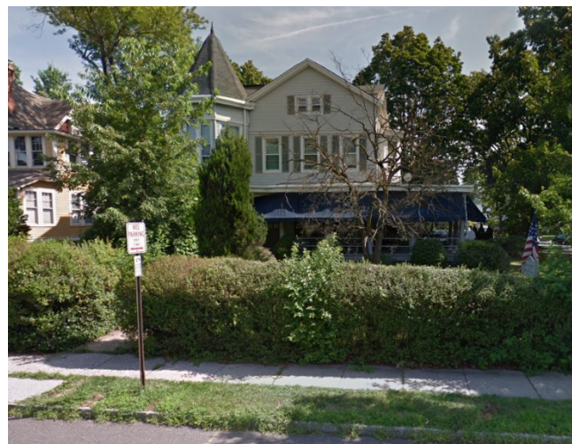
Figure 23: Essex Guest House at 271 Claremont Avenue.
