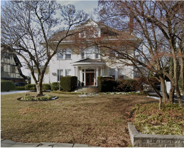
Figure 26: Walpan Manor at 176 Christopher Street.
