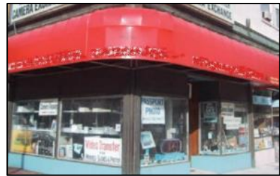
Figure 153 - NO - Do not allow signs to conceal or obscure historic building designs or detailing, such as an awning covering a historic transom.
