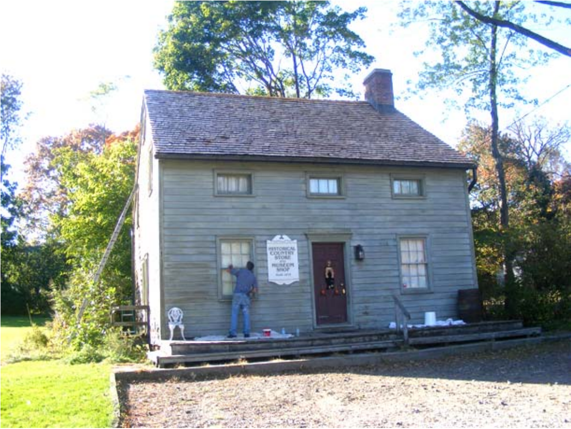
During exterior renovations, 2010
