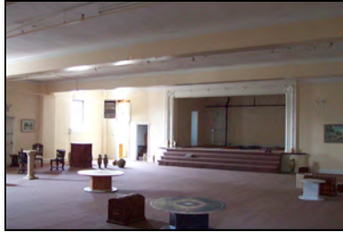
Figure 5.26: The second floor of 180 Bloomfield Avenue contains a large theater space needing renovations. The third floor is currently being used as a dance studio.
