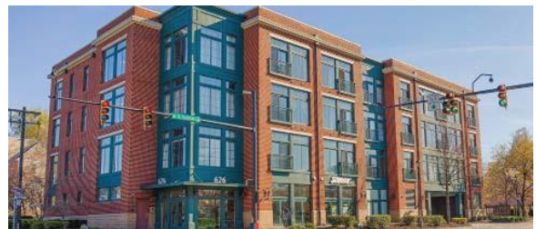
Figure 20: A recessed vertical bay element, similar in width to the building's standard bay, unobtrusively highlights the corner.
