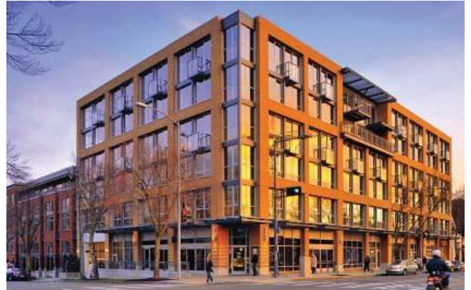
Figure 10: Borrowing from historic factory design and the modern office building, this interpretive Modern building uses traditional materials and a multi-layered façade to fit within its neighborhood, despite being larger and not relying on setbacks.
