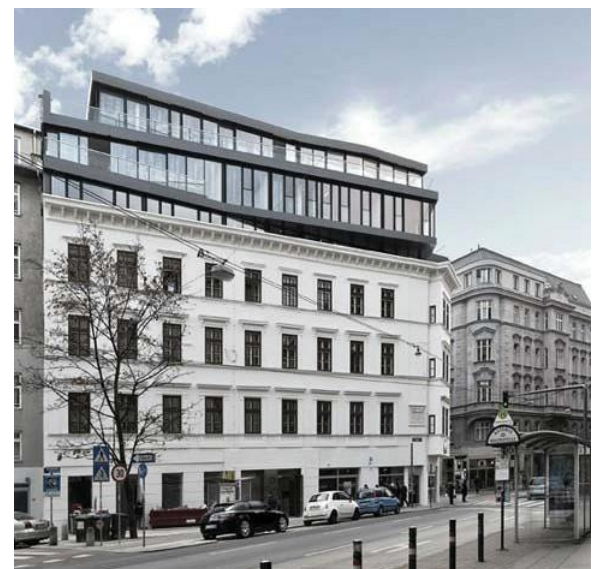
Figure 31: Skillful use of varying setbacks and tall bands of glass produce a dynamic new crown for a classical building.
