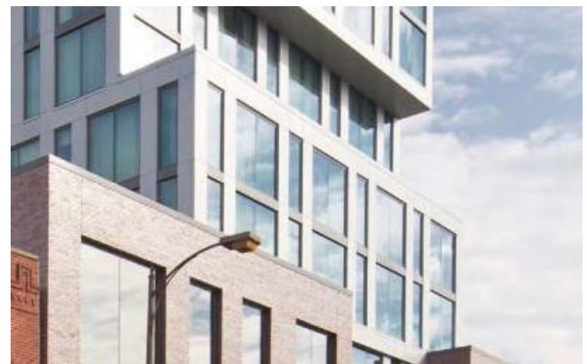
Figure 30: Relatively flat in appearance, the metallic finish applied to the upper story EIFS and the high ratio of void (glass) to solid (EIFS) produces a satisfactory “curtain wall” appearance, rather than the crudely detailed masses typically associated with EIFS.
