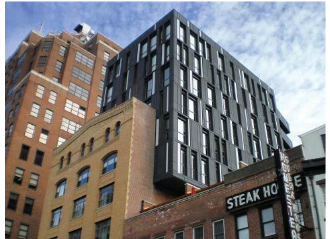
Figure 34: Inspired by its blocky neighbors with their punched openings, this addition steps back from the street, projects to the side, and uses metal as a contrasting material. It preserves its historic base while asserting its role in redefining the site's use from commercial to multi-family.
