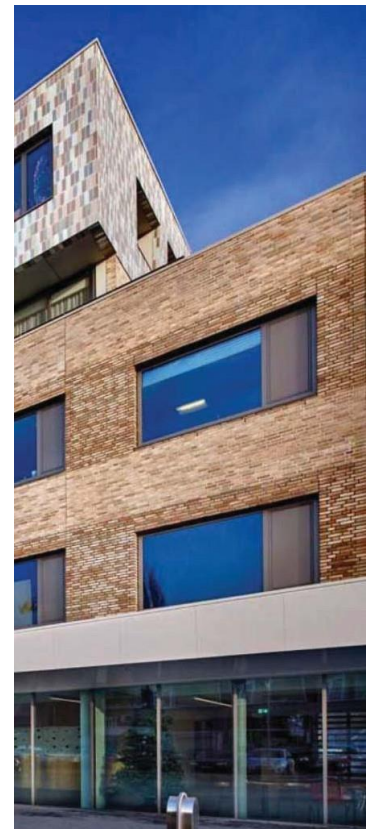
Figure 22: The base-middle-top composition of traditional "Main Street" facade design can be successfully reinterpreted to produce an effective midrise design.
