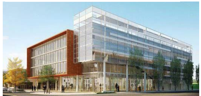
Figure 21: A single building, contrasting massing and materiality create the appearance of two structures meeting at a corner, each structure with its own apparent orientation and purpose. The open colonnade at the base helpfully unites the forms
