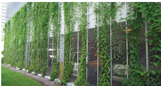
Figure 26: A "green" screen applied to a parking structure both shades the interior and softens the spaces around the deck.
