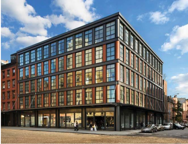
Figure 9: Holding the corner of a block in Tribeca, this transitional design borrows the proportions and materials of nearby historic cast iron buildings. In the middle floors, brick piers substitute for cast iron, a nod to adjacent masonry buildings.
