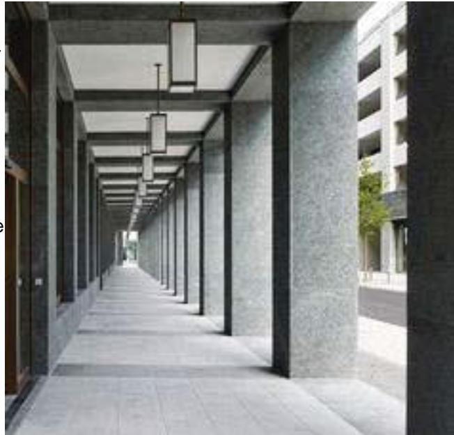
Figure 27: With a rhythm of simple masonry piers on both sides, this rectilinear loggia offers the same advantages as a classic arcade. Shallow recesses on one side can serve as art alcoves, promotional display, storefronts, or building entrances.
