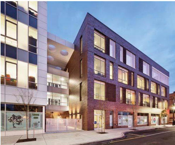
Figure 11: Historical material and style, such as brick and industrial openings, can be combined with new materials and expanded glazing to create a building suited for modern functions without seeming out of place in a walkable town center.
