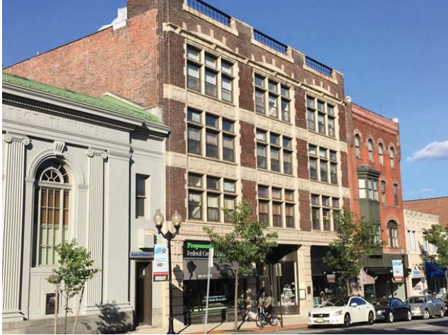
2.5.2-2: The Madison Building uses grids of varying scales and rhythms in order to reduce its perceived scale. Differences in height and width between it and its neighbors are visible in this photograph, but hardly apparent at the pedestrian level.
