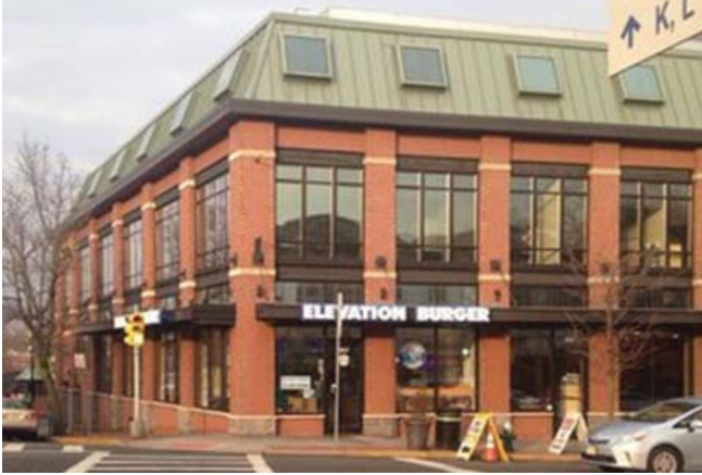
2.6-5: Buildings need not be Classical or Beaux-Arts style to be handsome, as 367 Bloomfield Avenue shows. Scale is controlled through tall brick pilasters, a bold steel canopy and a mansard roof concealing a third story.
