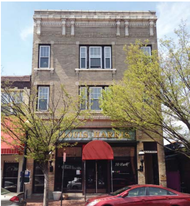
2.4.2-1: The Louis Harris Building on Park Street is organized into a bold bottom-middle-top composition using a tall storefront, decorative bands and individual ornaments. Windows are grouped and spaced to emphasize verticality.
