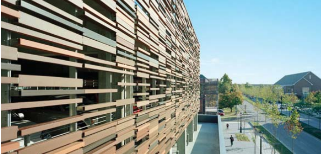
3.13-4: Permanent art can be integrated into the enclosure of a parking deck, providing lasting visual interest. In addition to the metal screen shown here, other options include decorative brick panels and mosaic panels (as at the Crescent Deck).
