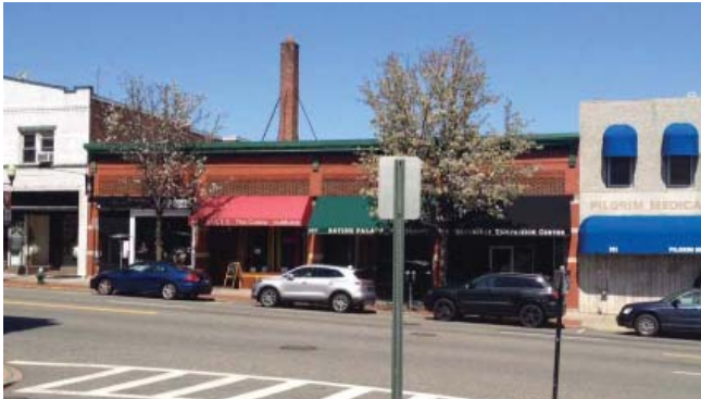
2.6-1: A simple single story building on Bloomfield Avenue, facing Seymour Street, is subdivided into bays by brick piers, emulating the storefront scale of the neighboring context.
