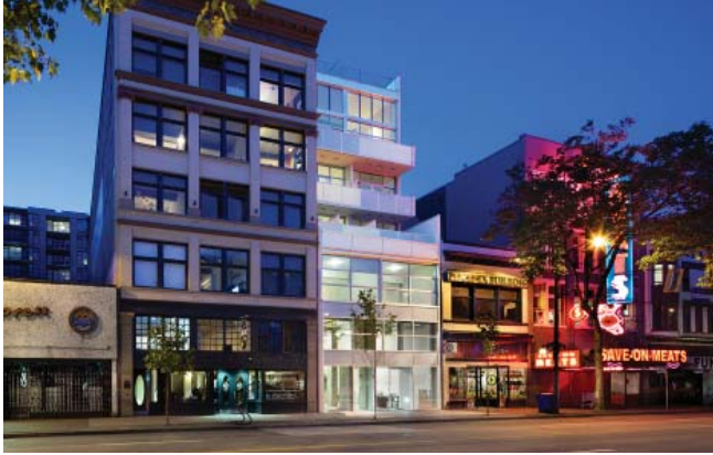
1.5-1: Encouraged: Carefully designed stepbacks in midrise buildings can produce matching rooflines between historic structures and larger, stylistically different neighbors. Buildings utilizing stepbacks are perceived as smaller by pedestrians.
