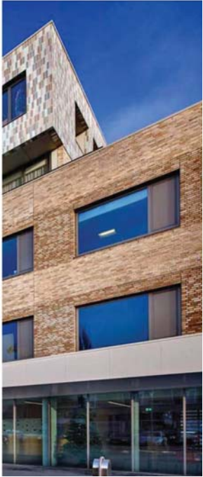
3.9-1: The base-middle-top composition of traditional "Main Street" facade design can be successfully reinterpreted in order to produce an effective midrise design.
