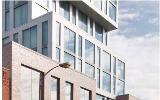
3.14-2: Relatively flat in appearance, the metallic finish applied to the upper story EIFS and the high ratio of void (glass) to solid (EIFS) produces a satisfactory "curtain wall" appearance, rather than the crudely detailed masses typically associated with EIFS.
