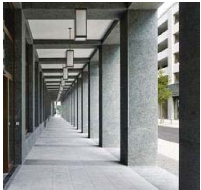
3.13-11: With a rhythm of simple masonry piers on both sides, this rectilinear loggia offers the same advantages as a classic arcade. Shallow recesses on one side can serve as art alcoves, promotional display, storefronts, or building entrances.
