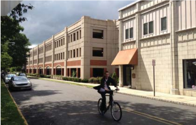
2.8-5: Along The Crescent, the Crescent Deck utilizes the architectural lessons from its commercial neighbors, extending the street-wall and emulating older architecture through modern precast concrete detailing.
