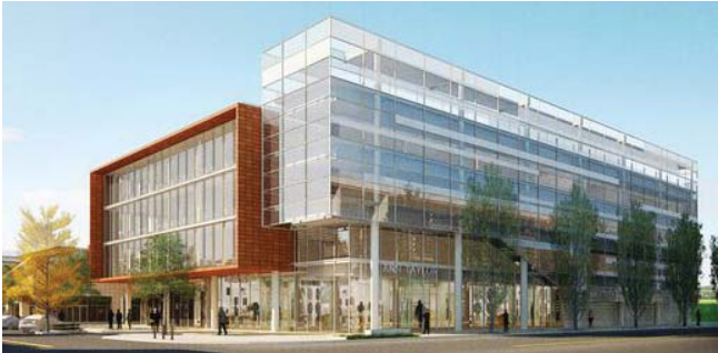
3.7-2: A single building, contrasting massing and materiality create the appearance of two structures meeting at a corner, each structure with its own apparent orientation and purpose. The open colonnade at the base helpfully unites the forms.
