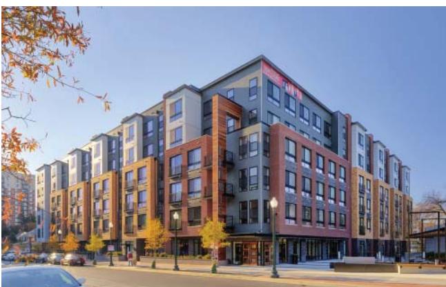
1.5-5: Discouraged: Over-prescription of stepbacks may backfire, creating unnecessary complexity at odds with most historic town center contexts. In this example, busy massing and minimally detailed surfaces emphasize bulk.
