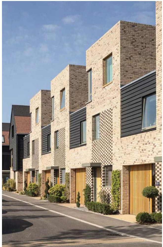
3.4-10: In lowrise construction, often used to transition from midrise masses to the scale of adjacent single family residences, smaller repeated masses are effective when articulated with materials and textures that echo traditional design.
