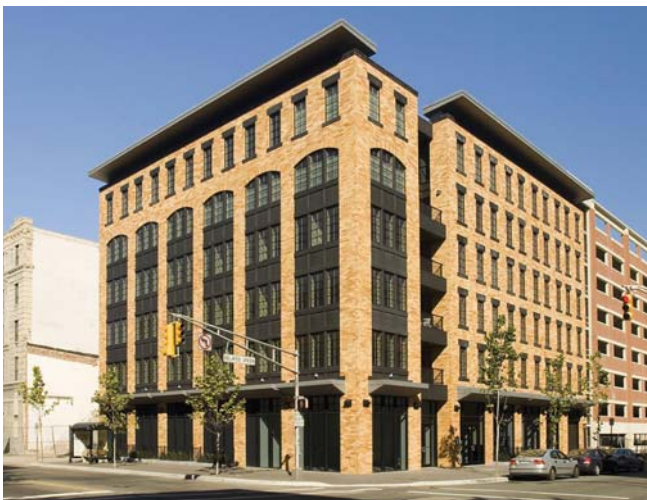
3.4-04: Consistent with the absence of stepbacks in historic midrise construction, this development uses a vertical gap on the side street to break one large mass into two. A simple palette of traditional materials balances an interpretive cornice.
