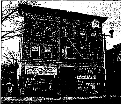
The Farrell Building 40-44 Valley Road Early 20 th Century Commercial
