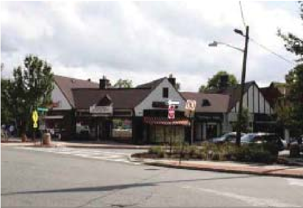
Figure 3.5.a: Key commercial building, designed by Clifford Wendhack
